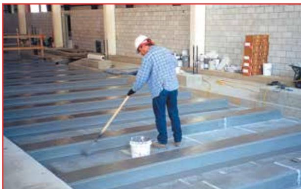
User-friendly **PENNCOAT™ Linings** and **PENNCOAT™ MR Linings** are practical and cost-effective solutions for secondary containment structures designed to resist occasional chemical splash and spill.
