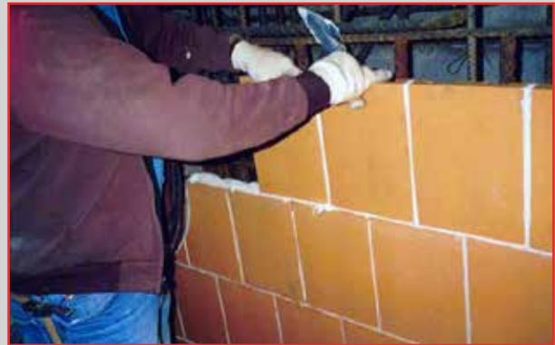
Vinyl ester mortars have historically been used in tile-lined, pulp bleach plant equipment. Our family of **vinyl ester PENNCHEM™ Mortars** provides customized performance to address variations in pH and temperature for optimal mortar longevity.
