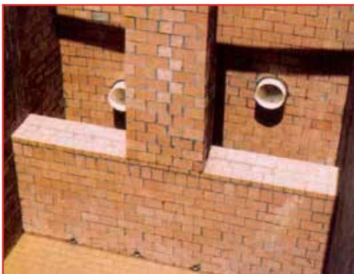
Though coatings have gained favor for their low initial cost, durable **acid brick linings** typically provide corrosion protection at a lower cost per year of service.
