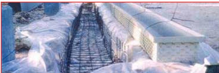
When downtime is critical, **shop-fabricated ACROLINE™ Systems trench and sump liners** save precious field construction time – concrete can be restored and lined in the same step.
