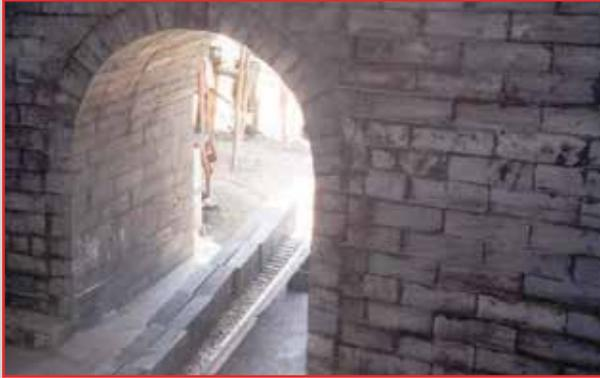
Phosphoric acid attack tanks are lined with **carbon brick** set in **FURALAC™ Green Panel Mortar** over a chemical-resistant membrane such as **TUFCEM™ II Membrane**.
