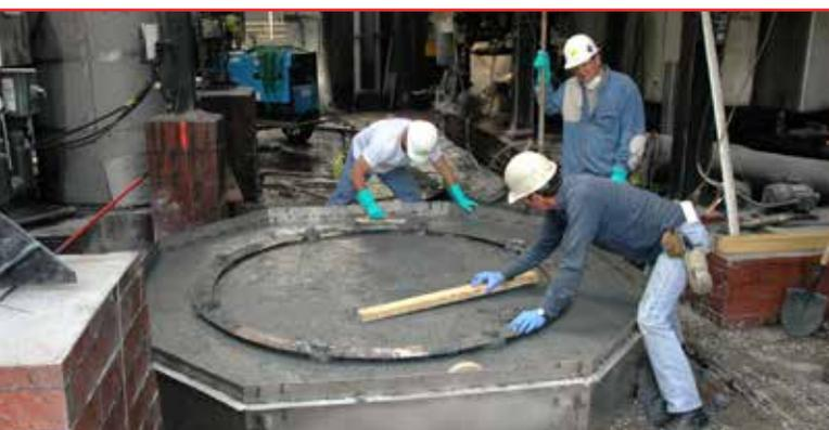
■ Leaking pump fluids can corrode Portland cement concrete pads from under base plates and mounting bolts. For structural support that is corrosion resistant, consider using **Corrosion Engineering polymer concrete**.
