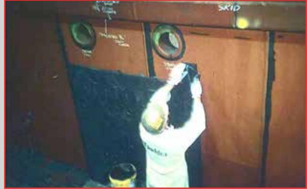
In acidic environments subject to thermal cycling, adding a layer of **PENNGUARD™ Block Lining System** behind the brickwork insulates the membrane and extends its service life.
