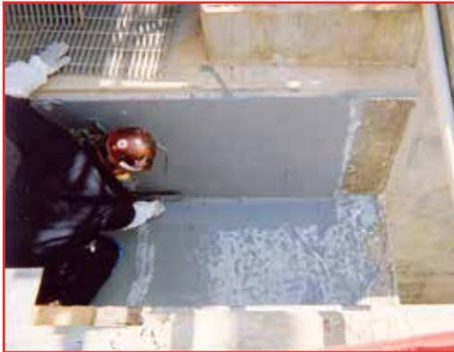
Durable fiberglass reinforced **PENNTROWEL™ MR and L/F Systems** can withstand constant chemical immersion and abrasion from sediment entrained in process effluent streams. The fabric also helps these linings maintain their integrity along inside corners, where seasonal thermal cycling could undermine a weaker lining system.
