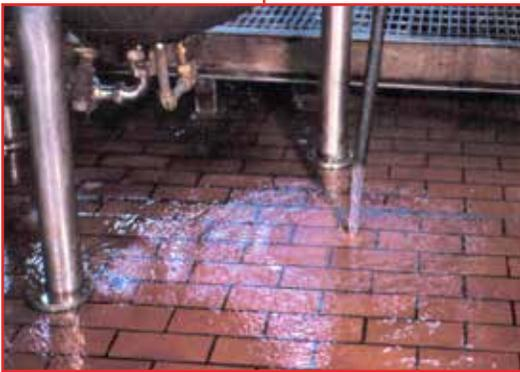
With unparalleled durability and thermal shock resistance, few alternatives outlast a properly specified, installed, and maintained **acid brick and membrane floor**.
